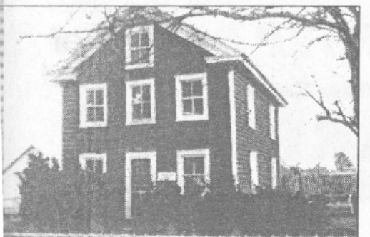
The "Down-the-island" School (1884?), 3842 Ridge Road.
